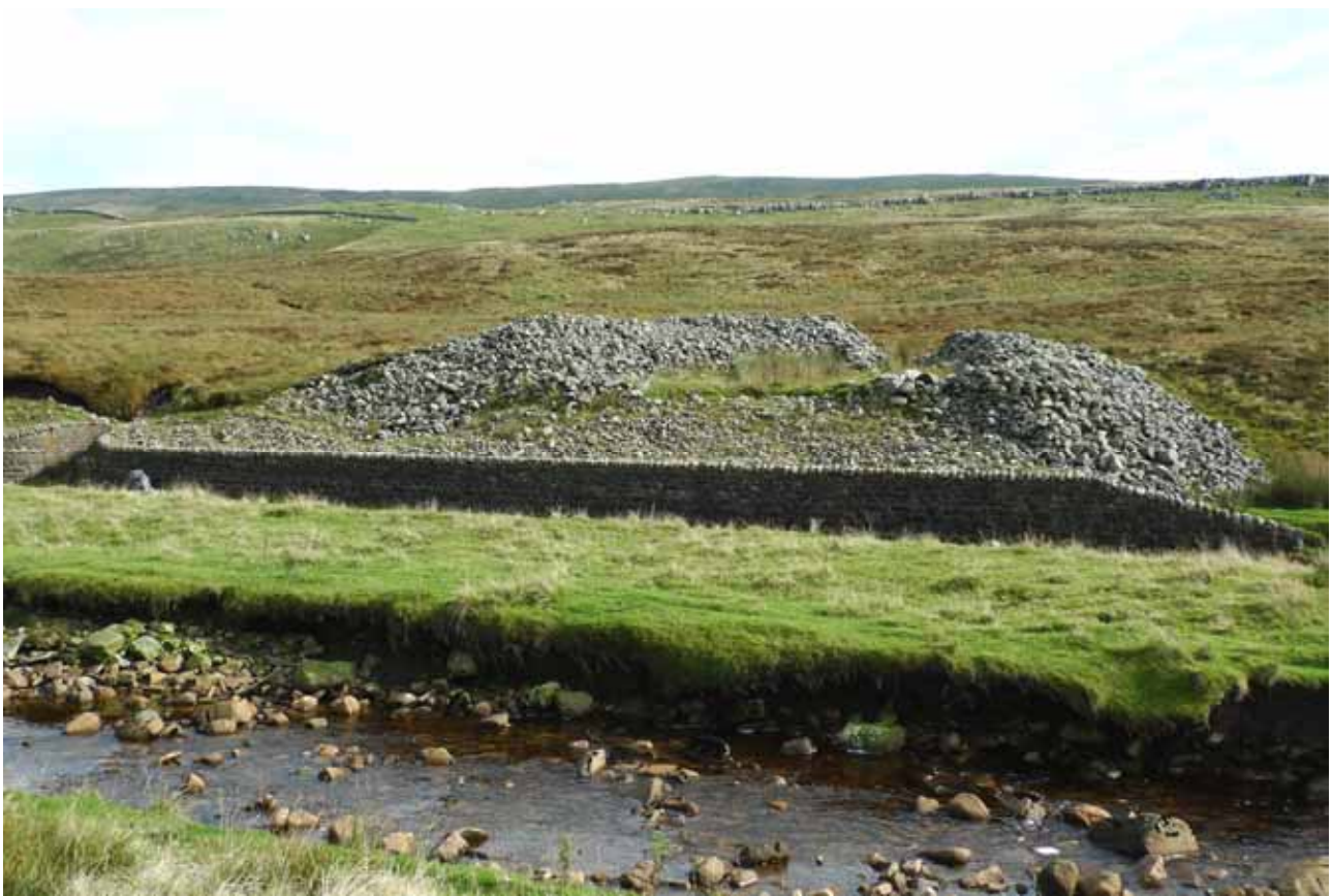
Plate 4 Feature 1 Apron full of Stones
